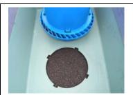
Insert the StormBasin cartridge down through the hole in the base of the unit. The colored ring on the cartridge should be facing upwards. Push the cartridge all the way through the hole until it rests on the bottom. Slowly turn the cartridge in a Clock-wise direction until the Tabs align with the slots and the cartridge body drops about ½ further down.
