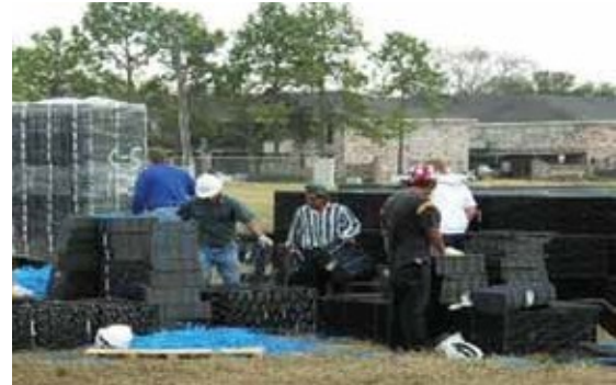
Figure 3: Assembling on site during excavation will increase speed once the excavation is completed
