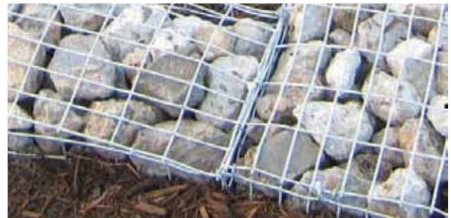
Figure 25: Overfill rock into gabion and seal tight to prevent sagging. Rock will settle over time.
