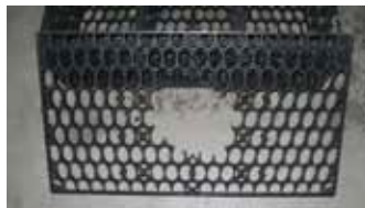
Figure 13 (Bottom): Place inspection port into underdrain module
