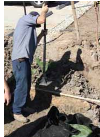
Figure 19: Compaction is critical in order to keep soils from settling around the tank.
