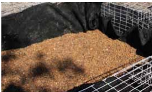
Figure 20 (Above): Place 6" of bridging stone on top of Biaxial Mesh
