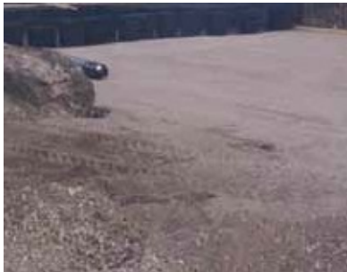
Figure 5: Base must be smooth to ensure units fit together without gaps
