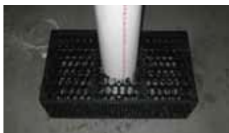
Figure 14 (Right): Cut inspection port to appropriate height stated on plans. Seal the opening on top of the pipe with the FocalPoint Inspection Port Cap or temporary lid
