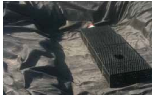
Figure 6: Rolled geotextile cut to fit the excavation is the most economical way to keep in-situ soils from migrating into the FocalPoint System. Geotextile strips must cover entire excavation.
