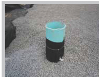
Fig. 17 Install port into R-Tank®.
