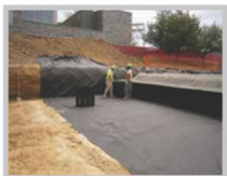
Fig. 5 Pull wrinkles out of geotextiles so material lays flat.
