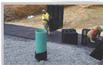
Fig. 11 Installed Inspection Port
