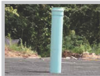
Fig. 16 Installed maintenance port
