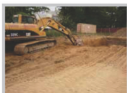
Fig. 4 Excavate according to plans, following all governmental regulations.
