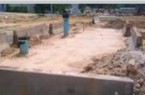
Fig. 28 Secured R-Tank® installation using Jersey Barriers.
