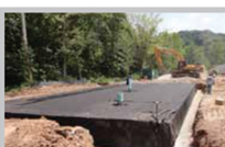
Fig. 21 Finished envelope should lay flat against R-Tank®.
