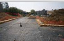
Fig. 25 Overlap Geogrid 18" or as required by plans.
