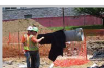
Fig. 22 Seal the pipe boot with the included band clamps and duct tape.
