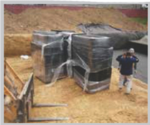
Fig. 3 Installation can be sped up by either assembling the tanks in the excavation or placing the pre-assembled tanks in the excavation.
