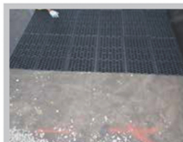
Fig. 18 Maintain 12" overlap on textile.
