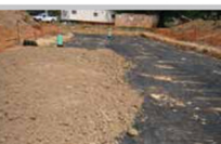
Fig. 26 Pushing backfill parallel to the Geogrid prevents the grid from shoving.
