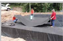
Fig. 20 Encapsulate R-Tanks® with geotextile.
