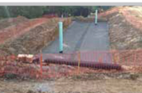
Fig. 27 Secure the installation with temporary fencing.
