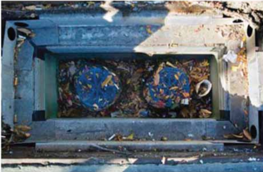
The inserts remove heavy metals, sediment, bacteria, organics, nitrates and litter from storm runoff.
