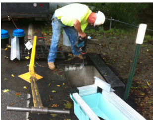
Stormdrain retrofit with StormBasin in Hilltop Beach Area
