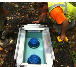
StormBasin retrofit in Lake Oscawana Watershed
