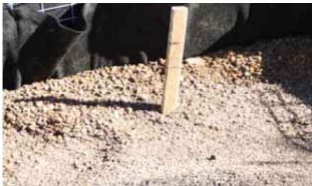
Figure 22: Place Element 1 soils, being careful not to mix with any other site soils, to specified depth
