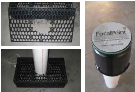
Figure 13 (Bottom): Place inspection port into underdrain module
