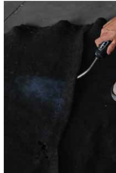
Figure 29: Geotextile being melted together with a torch.
