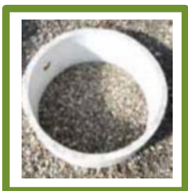
Figure 4: Pipe Installed Into Media
