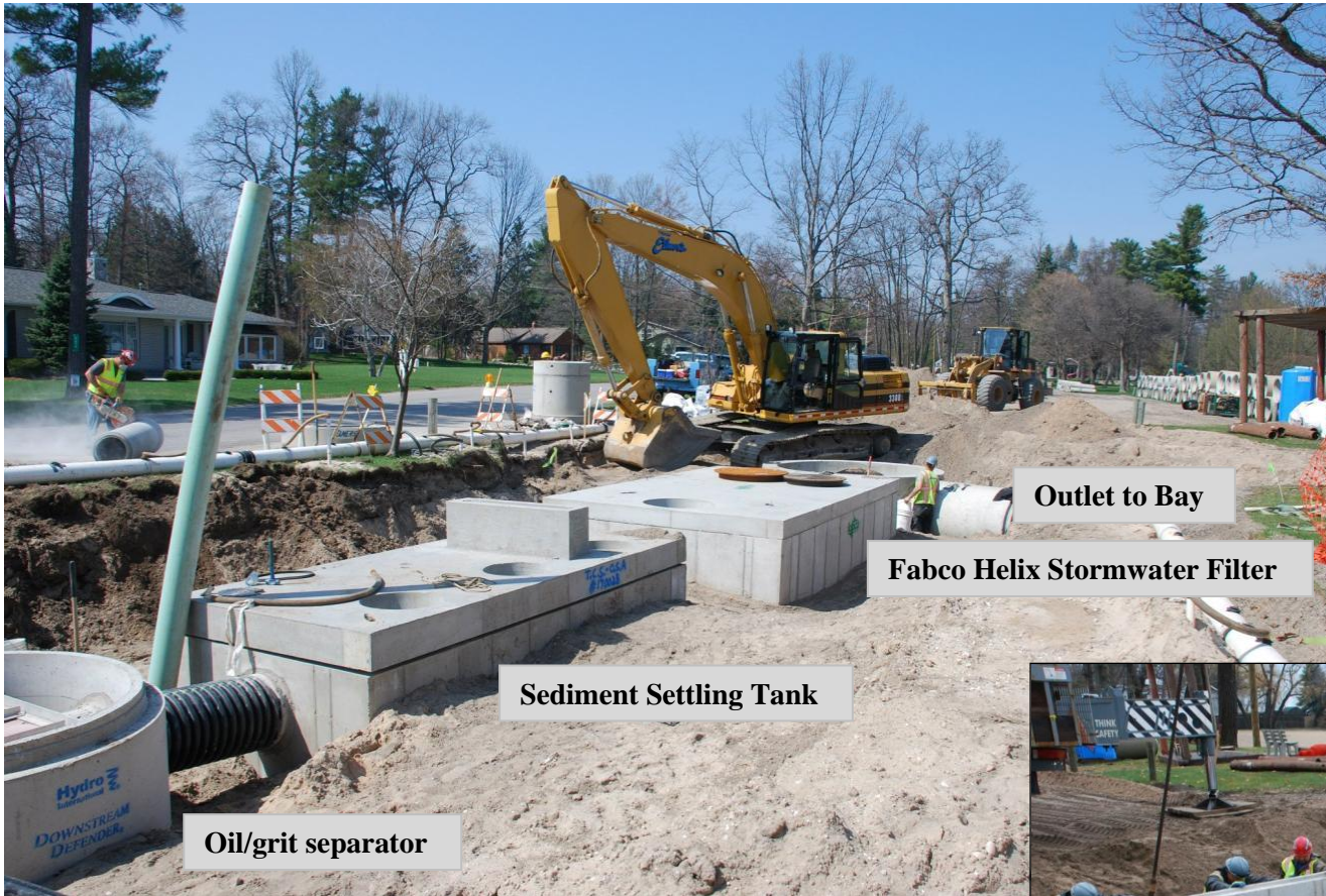
Left: Stormwater filtration treatment system installed, south end of East Bay Park
