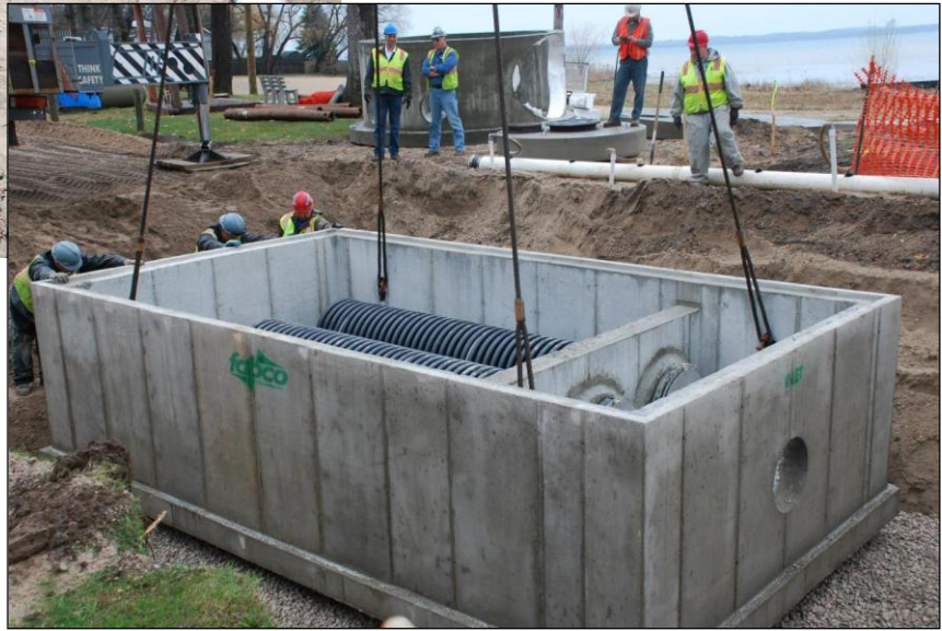
Above and Left: Fabco Helix Filter installation
